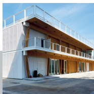
BUSINESS AREA LAVORI
